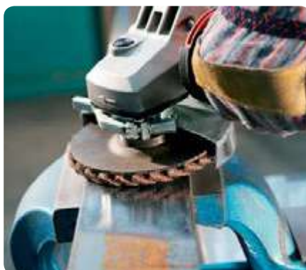
Professional derusting and descaling
